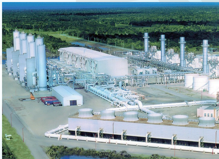
Nitrogen and oxygen are separated from liquid air in this fractional distillation plant
