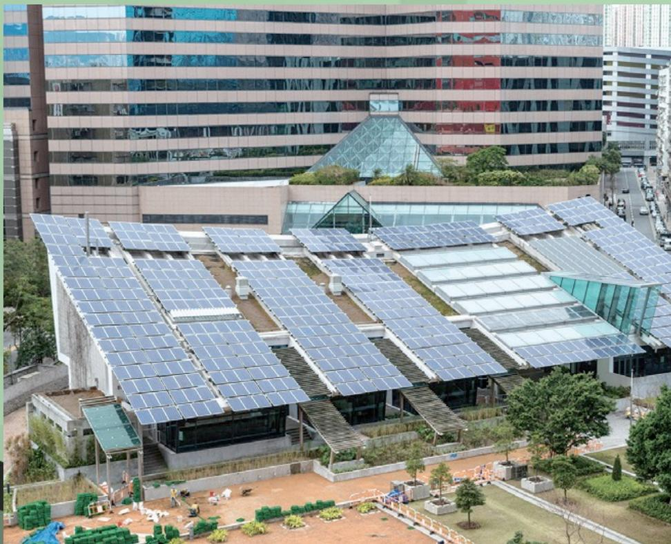
The Zero Carbon Building in Kowloon Bay generates on-site renewable energy from photovoltaic panels and a tri-generation system using biofuel made of waste cooking oil
